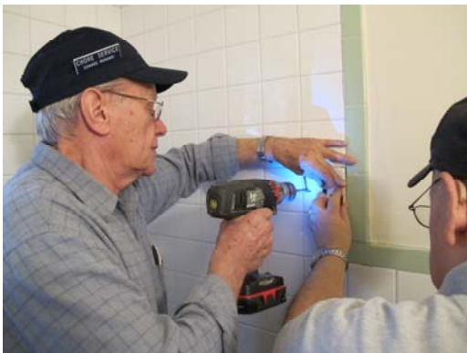
Crew chief Ed Morandi prepares to install a grab bar. Chore volunteers do simple repairs that keep seniors and people with disabilities safe in their homes.
